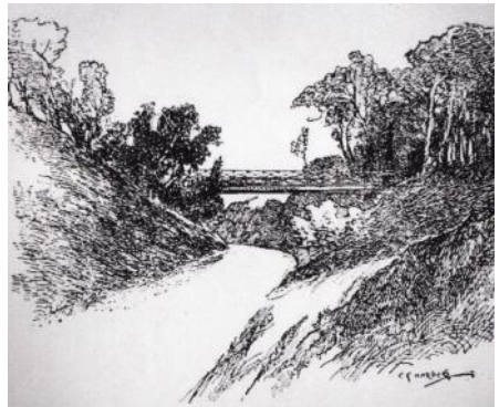
The Suspension Bridge, Reigate Hill 1892
